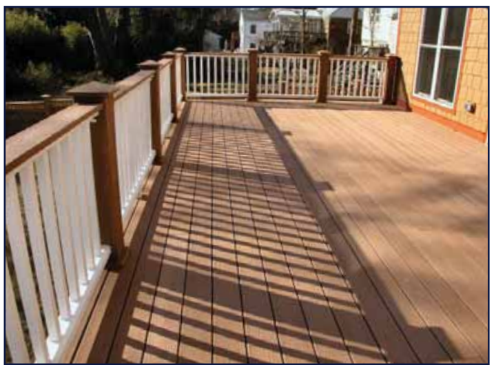
Deck off Living Room
